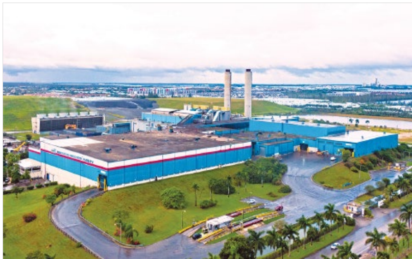
Picture 4. Miami Dade Resource Recovery Facility by Miami Today News
