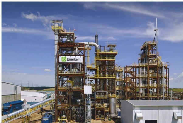
Picture 6. Enerkem Alberta Biofuels Facility by Enerkem
