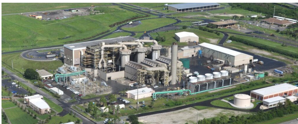
Picture 2. Pinellas County WTE Facility by Pinellas County
